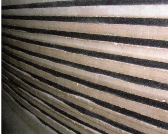
Foam Inserts Installed in Pavement
