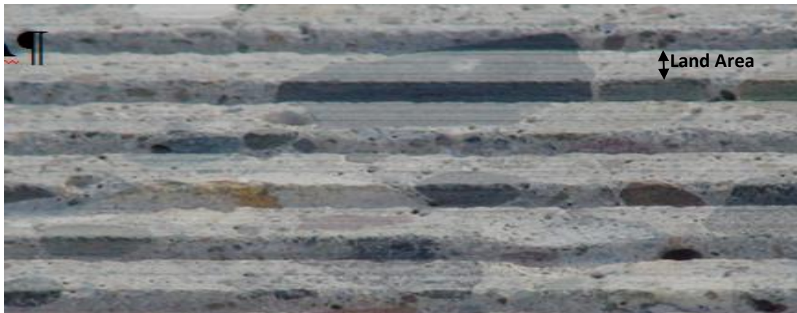
Figure 10- Photo of Purdue Negative Texture Profile (e.g. NGCS) and Land Area
