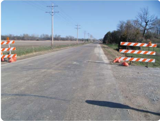
North First Street before the concrete overlay.
