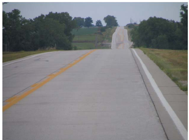
This stretch of 50+ years old pavement looks great, and is still serving Nebraska residents admirably. How many other kinds of surfaces see 50 years before needing major repair?
