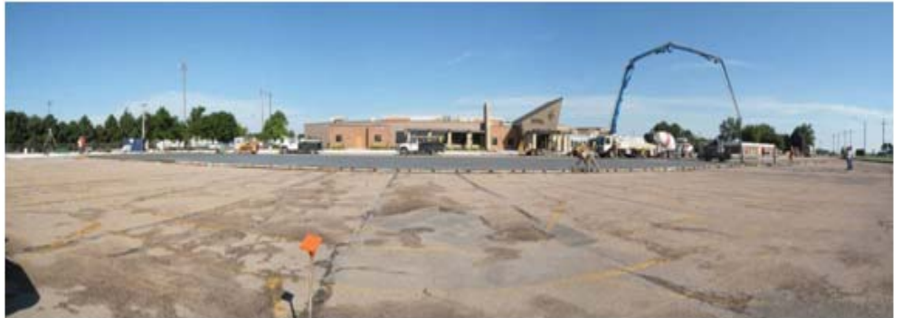
Looking northwest at Northwest High School while pouring the concrete overlay.
